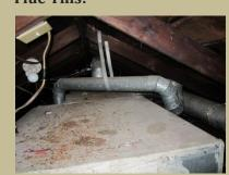
Furnace flues should always slope upwards. This was scary!
