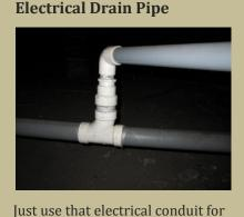
Just use that electrical conduit for drain lines. Yeah that will work!
