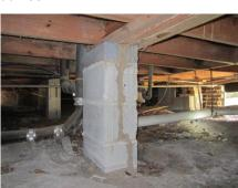
damage to the subflooring under the bathroom area. The most interesting discovery in the crawl space was the termite tubes present on the interior piers and the floor joists.
