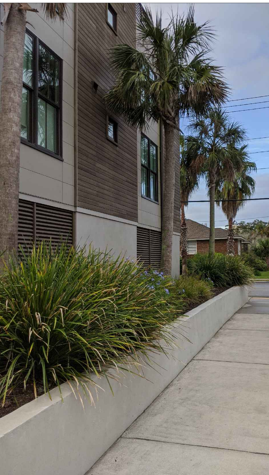
PERIMETER RETAINING WALL
