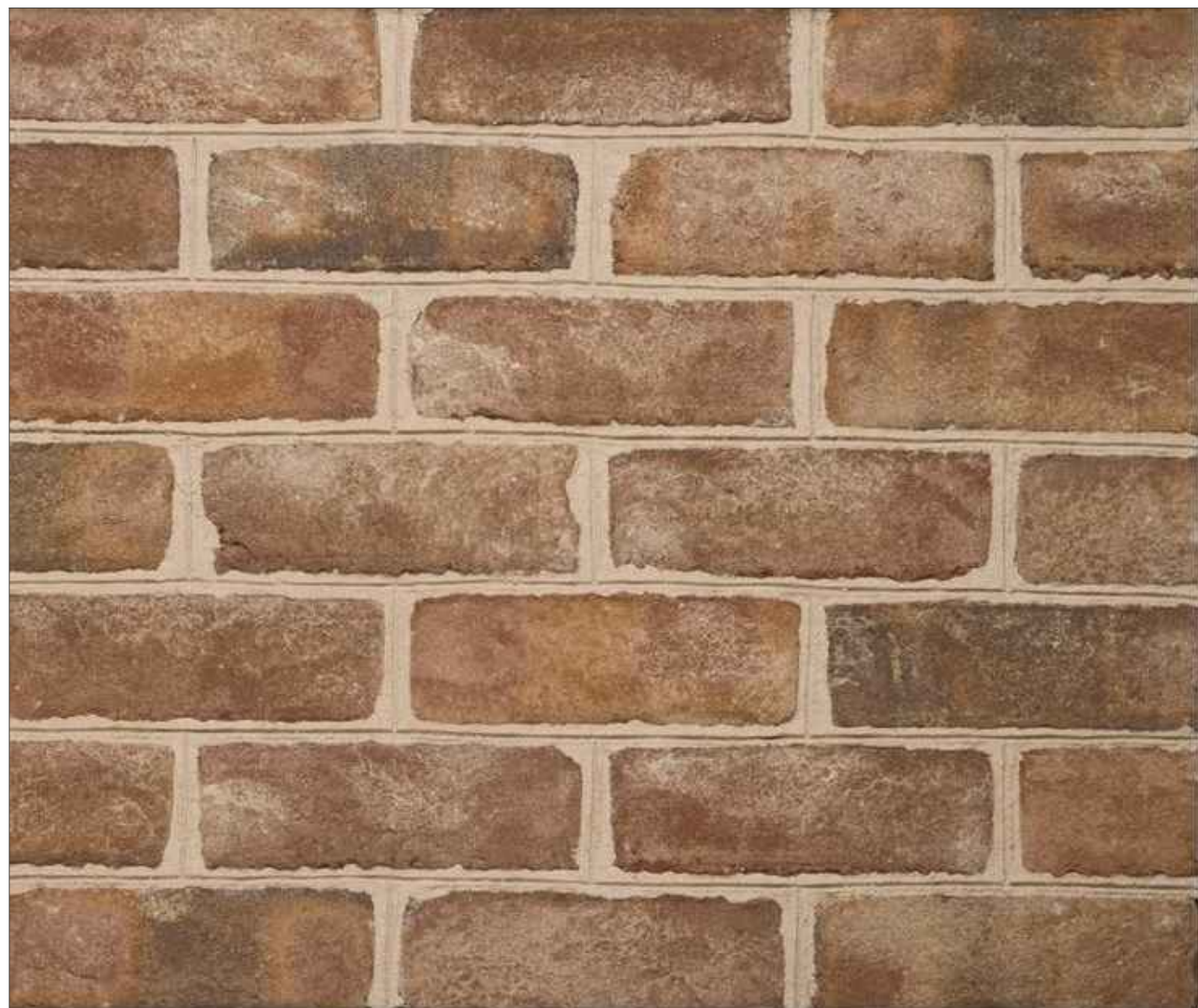
OLD CAROLINA BRICK (CHIMNEY, FRONT STEPS, LANDINGS)
