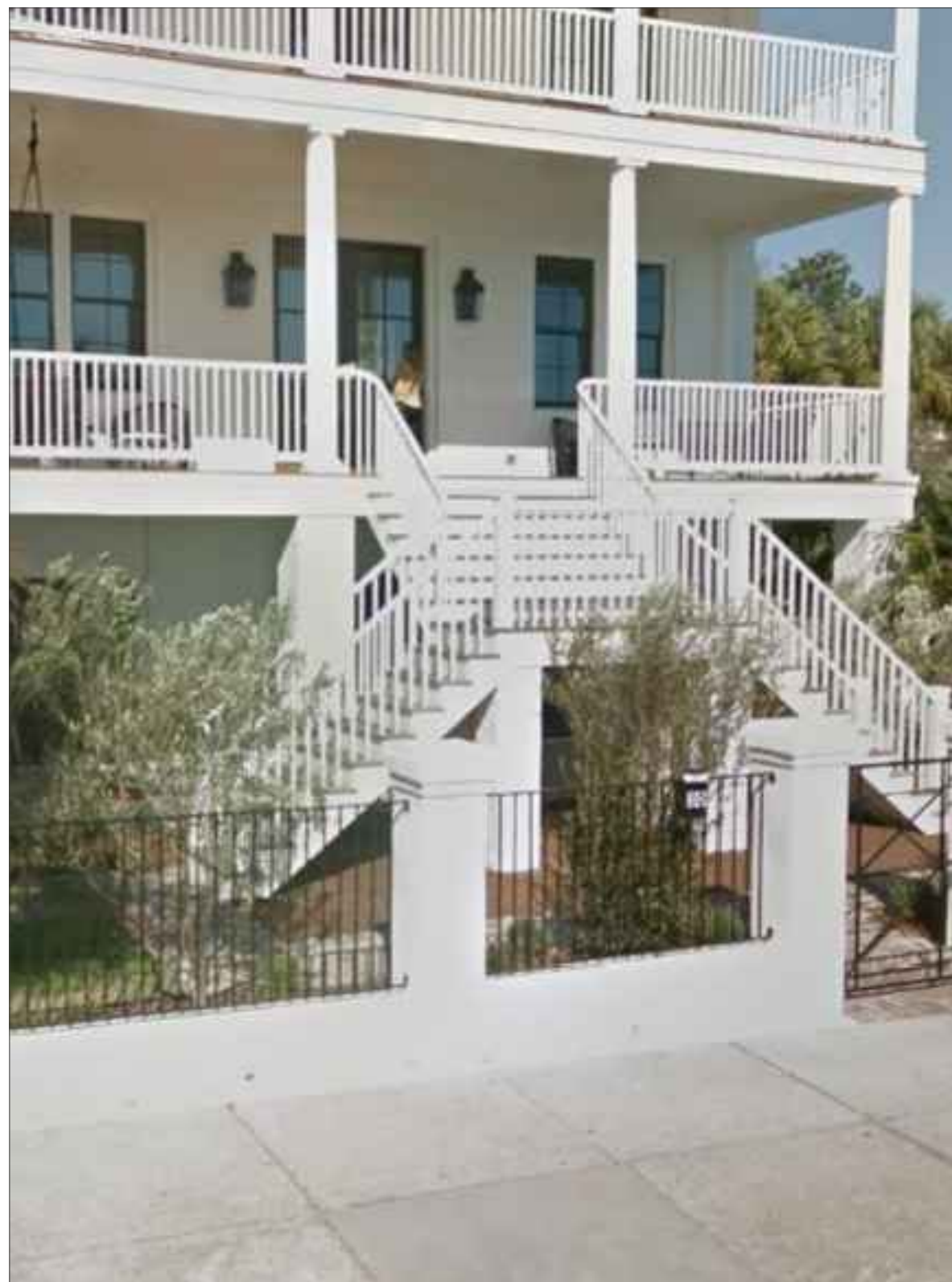
MIRRORED ENTRY STAIR
